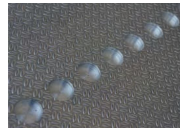
Lashing attachment in the floor
