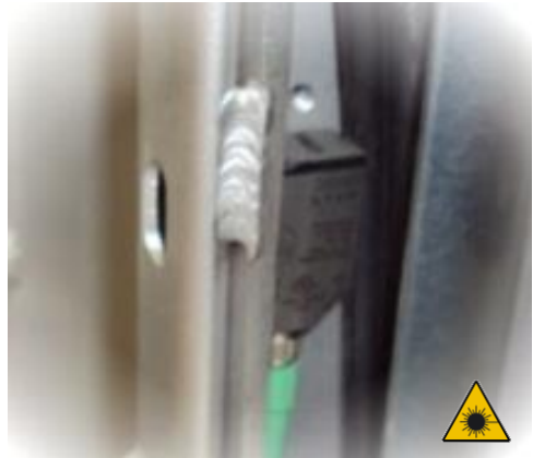
Closing obstacle detection cells located in the door risers. (about 6 cm above the threshold)
